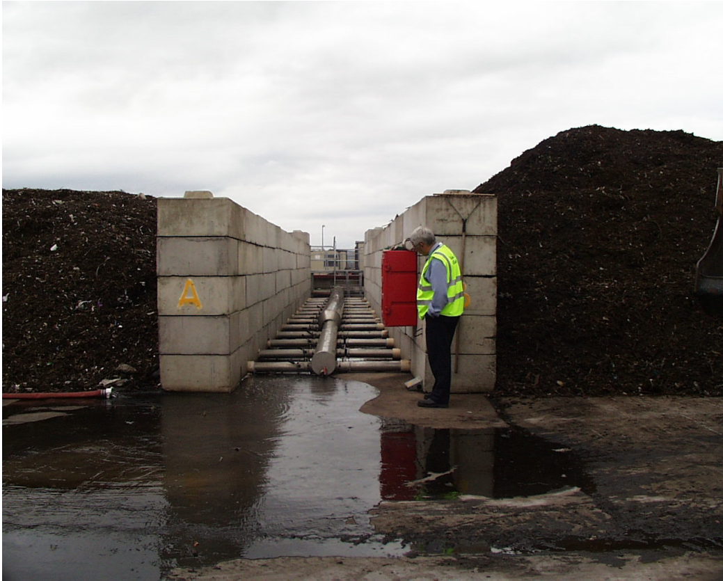
A VAR Aerated Static Pile at Sandy Road Composting Facility, Galway, Ireland
